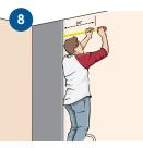
the next vertical strip of double-sided tape, centered on the 24" mark. Again, do not remove the protective covering. Apply tape horizontally at the ceiling and the floor as you did in step 7. Keep protective covering on tape. NOTE: Walls can be imperfect so measure for each sheet of wall covering to ensure proper fit.
