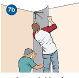
go. NOTE: Half of the outermost strip of vertical tape should remain exposed for the next sheet to be adhered.
