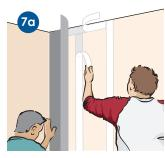
Now remove the protective layer from the other strips of tape. Carefully adhere the wall covering to the tape, smoothing as you
