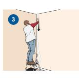
4. Measure 24" from the corner of the wall. Mark the wall in several placed from the top of the wall to the bottom.
